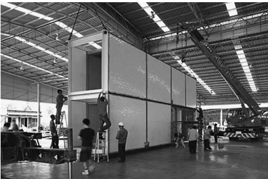
3.12 Pre-manufactured Modular Housing Units, Japan, 2011. Photo: Yasutaka Yoshimura Architects
