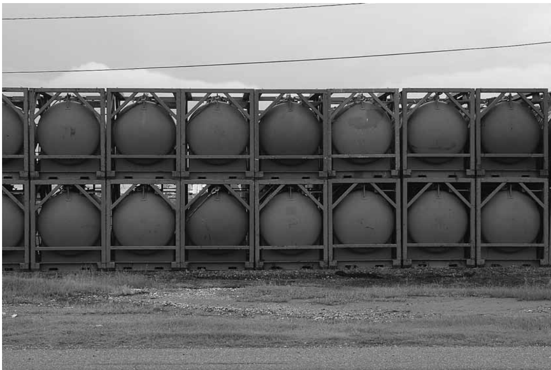
3.10 Propane Tank Rack, BP Floatel Encampment, 2010. Photo: S. Verderber
