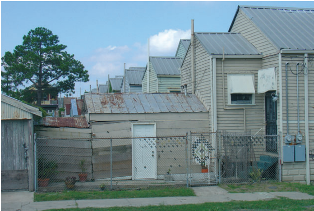
5. Shotgun side/rear profile, Bayou St. John Neighborhood, depicting telescopic kitchens, narrowly proportioned yards, and storage sheds in a city where basements are not possible. (Photo by author.)
